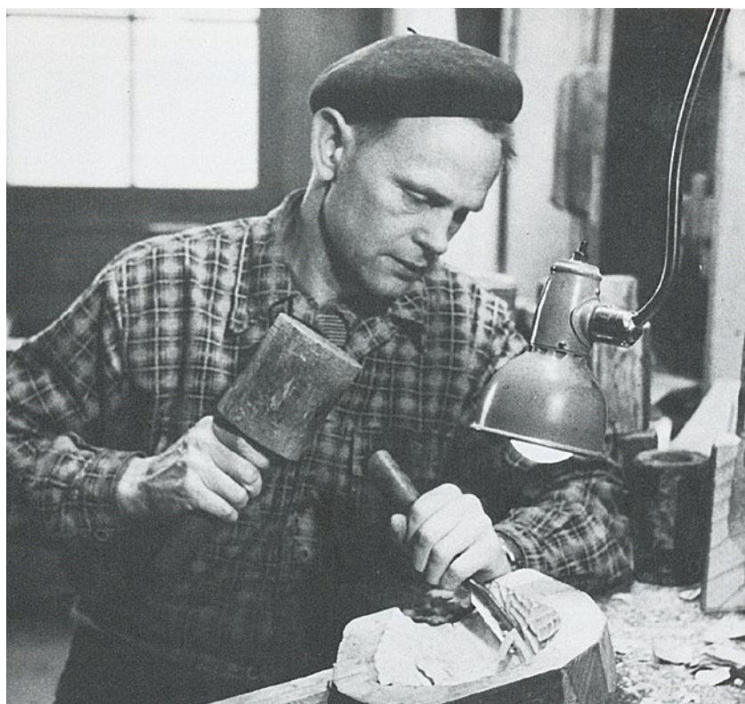
At Boda glassworks in the 1950s, mould maker Börje Franzén made all the graphite and wooden moulds, for various artists including Erik Höglund. Photo: Henrik Hultgren, 1954, The Glass Factory archive.
