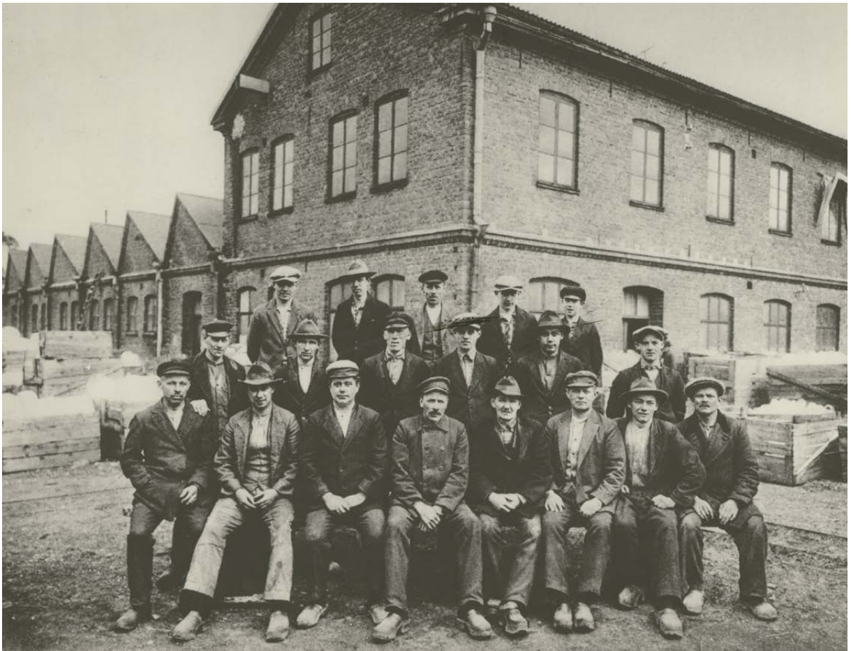
Group picture in front of the cutting workshop at Pukeberg's glassworks in 1918. The saw-toothed roof with windows on the shorter sides was built to let a lot of light into the workrooms. This type of roof has also become a symbol for the term "industry" Photo: KLM archive.
